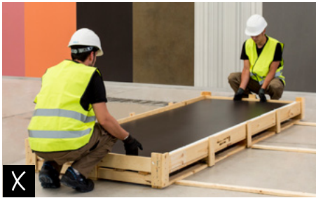
Do not position yourself opposite your workmate to remove the ceramic slabs from the box.
