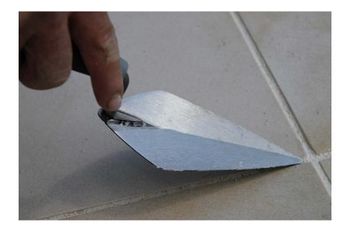
Allow the pointing to cure for 15 minutes prior to trowelling off. After 15 minutes use a trowel or pointing tool to compress the pointing mix into the joint.
