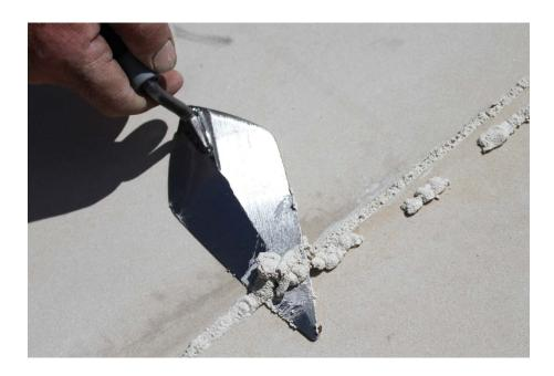
15 minutes after the pointing mix has been trowelled any excess pointing mixture must now be removed. Using the trowel, now scrape off any excess mortar and discard.
