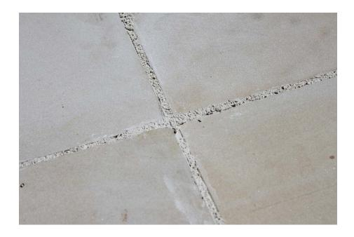
Once you have completed all the pointing you should allow ample time for the pointing mix to cure. Avoid allowing any kind of traffic (foot or vehicles) on the pointed area for a minimum of 24 hours (this process could take longer in periods of colder weather).
