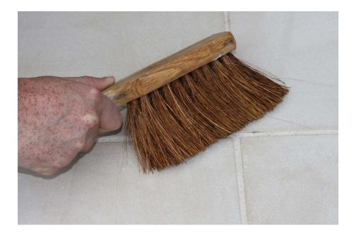
Now leave the pointing mix to cure for a further 15 minutes. Any excess pointing mix should now be carefully brushed off. Using a soft brush carefully brush the surface of the paving to remove any further excesss pointing material.
