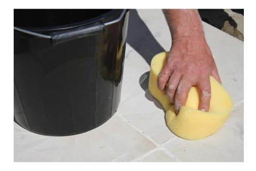
Spills and smudges of the pointing mix are a common occurence of this process and are very difficult to remove once the pointing mix has cured. Any stains should be quickly removed before they have had time to cure. This can be done easily. Using a sponge and bucket of clean water wipe off any excess pointing mix or stains from the edges of the pavers.
