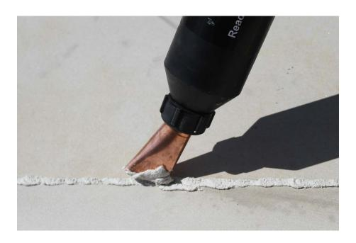
It is very important to work in small areas allowing yourself sufficient time to complete the pointing process. Once you have completed a small area of pointing you should now follow the same procedure until the whole area has been pointed.
