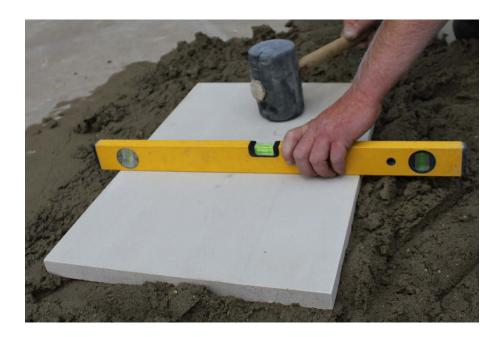
Take some semi-wet mortar and spread out a full bed, slightly larger than the first paver to be laid. Using a trowel, create peaks and troughs in the mortar. Place the paver on top of the mortar. At this point, the paver should be sitting higher than the string lines. Using a rubber mallet, tap the paver down until it aligns with the strings. The paver should be level along one plane and sloping on the other plane. Confirm this using a spirit level.
