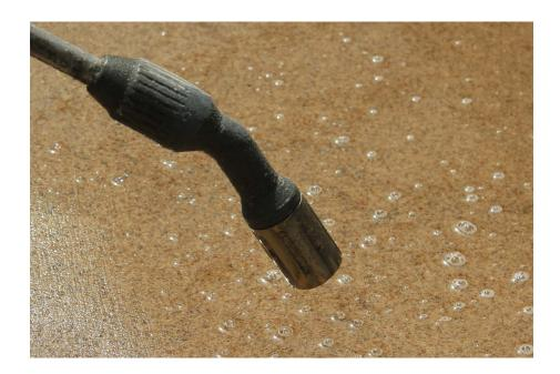
Using a low pressure sprayer apply a generous 1st coat of sealant. Be sure to apply across the complete surface of the stone and working in even lines across the paved area from left to right. Under no circumstances seal the backs or sides of the slabs (unless side is exposed on step tread or coping). Sealing the undersides and sides of slabs will compromise the adhesion between the bedding layer and jointing material.
