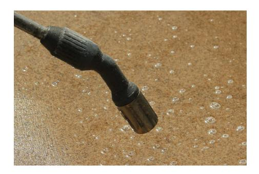
Using a low pressure sprayer apply a generous 2nd coat of sealant. Be sure to apply across the complete surface of the stone. Work in even lines at 90 degree angle to the direction of the first coat to ensure full coverage. Under no circumstances seal the backs or sides of the slabs (unless side is exposed on step tread or coping). Sealing the undersides and sides of slabs will compromise the adhesion between the bedding layer and jointing material.
