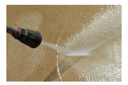
Stone must be clean and clear of any debris prior to any sealing work being undertaken. London Stone advise that the stone is brushed to remove any loose debris and then thoroughly cleaned with a pressure washer.
