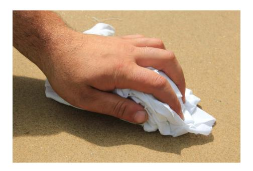
It is essential that excess sealant or pooling is removed from the surface of the natural stone before it dries. You must thoroughly remove any excess sealant at this point with a clean white cloth. Excess sealant will leave unsightly marks if not removed. Stone may need to be cleaned & dried again if you do not apply the second coat immediately.
