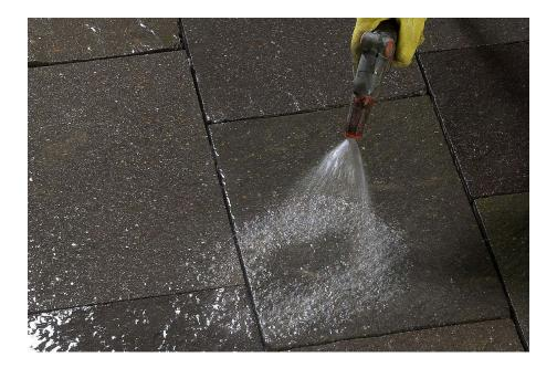
Clean the surface and joints of all dirt, detritus, cement residues and any other contaminants. Ensure that the joints are cleaned out to the required depth.
