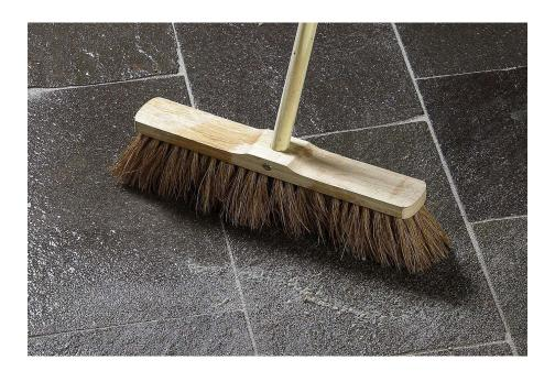
Finally, remove any remaining fine residues with a damp coconut fibre brush. Do not brush the dry residual material into unfilled joints. Clean the brush frequently with fresh water. Ensure that residues are completely removed.
