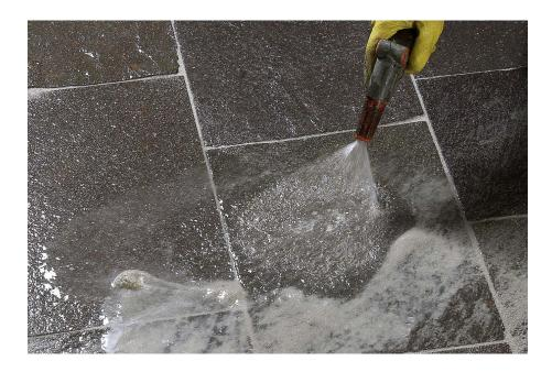
After about 5 minutes, or immediately in temperatures higher than 15°C, remove any excess mortar completely by spraying lightly with water from a hose at a distance of approximately 25cm. Avoid washing out the joints. Be careful to clean the paved surface towards areas not yet jointed and do not allow any water containing residues to pond, stand, dry out or run off over completed areas.
