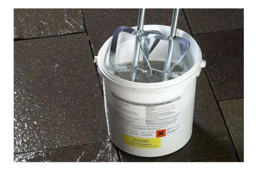
Using a drill with twin spherical mixing paddles, mix the resin coated aggregate (component A) materials together and then add the liquid hardener (component B) until a smooth, homogeneous consistency is achieved. Do not add any water to the mix and do not use any material that is not thoroughly mixed.
