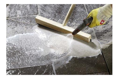
Pour the mortar directly onto the pre-wetted paving surface. Work thoroughly into the joints using a rubber squeegee whilst spraying lightly with water from a hose, ensuring that all voids are well packed. The product will be very free flowing. Work from the highest point of the paving to the lowest. Ensure that the paving stays fully wetted throughout application.
