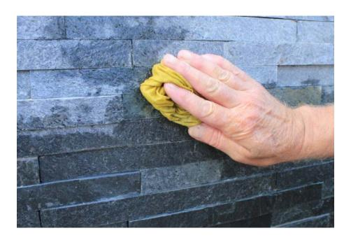
Adhesive spills are a common occurrence when installing natural stone cladding. Always keep a bucket of clean water and a cloth close to hand and remove any spills immediately.
