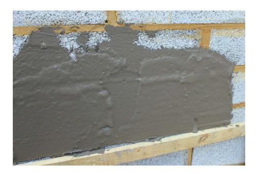
Cladding should be ixed to the wall using a flexible, rapid setting exterior adhesive. Using a tiling trowel, evenly butter the surface of the wall with the adhesive and irmly press the tile to the wall. Check that the cladding is horizontally level using a spirit level. Using a trowel, scrape off any excess adhesive.
