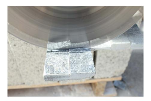
The cladding is supplied in Z shape interlocking format to provide a strong bond. The left hand Z will need to be cut off the cladding to enable the left hand edge of the cladding to be flush with the left hand edge of the wall.
