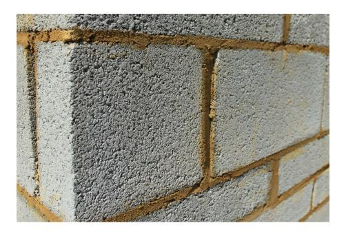
Good preparation is key to the success of any successful natural stone installation. Walls to be cladded should be constructed using concrete blocks and built on top of strong concrete foundations. Walls should also be flat and free of any protruding mortar. If possible try and design the wall to dimensions that minimise the number of cuts to be made to the cladding
