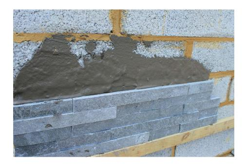
Install the remainder of the cladding as described previously. Regularly check the levels of the cladding using a spirit level. Small plastic packers may sometime be required to maintain an even level of cladding across the courses.
