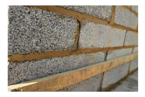
Prior to fixing the first course of cladding to the wall you should fix a level timber baton across the length of the wall. The top of the timber baton should be set at the same height as the underside of the first course of cladding. This is done to prevent vertical migration of the cladding before the adhesive has had a chance to set.
