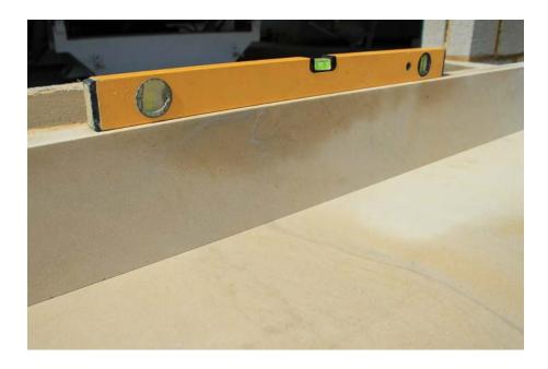
The riser should sit directly on top of the step tread with no gap between the top of the step tread and the bottom of the riser. Butter the back of the riser with the same mortar mix as used to lay the step tread with. Firmly press the riser against the step base. Using a small spirit level check that the riser is level vertically and using a tape measure check that riser is square to the step tread that it sits upon.
