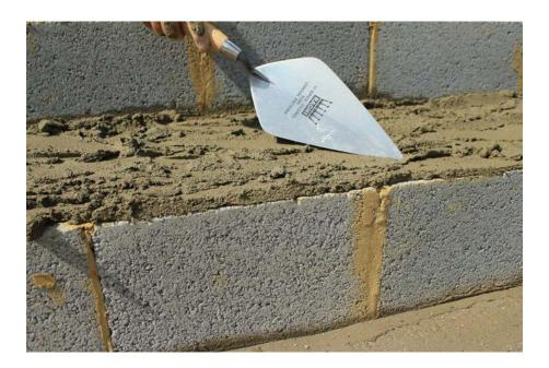
Spread a layer of mortar across the base where the first step tread is to be fixed. The mortar bed should be approximately 20-25mm thick. Use a trowel to create peaks and troughs in the mortar bed. For extra adhesion the back of the coping stones should be painted with an SBR & cement slurry.
