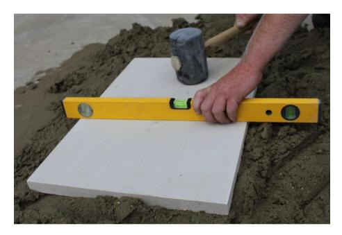
Take some semi-wet mortar and spread out a full bed, slightly larger than the first paver to be laid. Using a trowel, create peaks and troughs in the mortar. Place the paver on top of the mortar. At this point, the paver should be sitting higher than the string lines. Using a rubber mallet, tap the paver down until it aligns with the strings. The paver should be level along one plane and sloping on the other plane. Confirm this using a spirit level.
