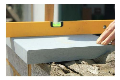
Lay your first coping stone onto the mortar bed and using a rubber mallet and spirit level; tap the coping stone down to the desired level. The coping stone should be horizontally level. A small fall should be incorporated back to front to aid water run off (This step is not required with weathered coping stones). Using a tape measure, check that the coping stone is square to the wall.
