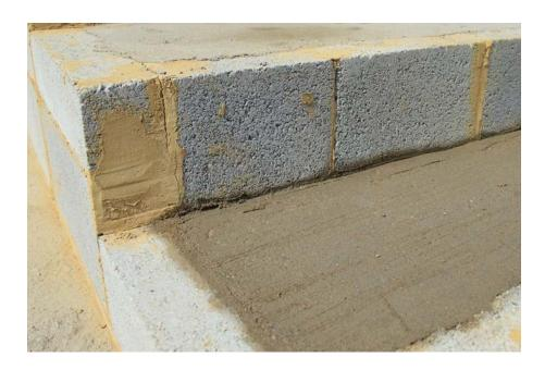
Good preparation is key to the success of any successful bespoke stone steps installation. Step bases should be constructed using concrete blocks and built on top of strong concrete foundations. Step bases should also be flat and free of any protruding mortar. If possible try and design the step base to dimensions that minimise the number of cuts to be made to the steps. Any cavities should be filled with concrete or compacted DPT (MOT) Type 1.
