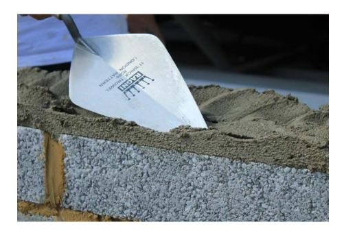
Spread a layer of mortar across the base where the first coping stone is to be fixed. The mortar bed should be approximitely 10-20mm thick. Use a trowel to create peaks and troughs in the mortar bed. For extra adhesion the back of the coping stones should be painted with an SBR & cement slurry.
