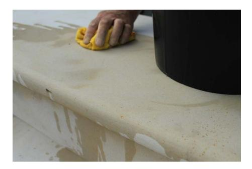
Using the techniques as described above, continue to lay all the step treads and risers until complete. Be sure to continually check the levels with a spirit level. Mortar spills can be a common occurrence during step installation. Have a bucket of clean water and sponge close to hand and clean up any mortar spills immediately as they happen
