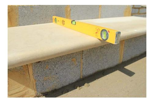
Lay your first step tread onto the mortar bed and using a rubber mallet and spirit level, tap the step tread down to the desired level. The step should be level from left to right and a small fall should be incorporated from back to front to aid water run-off.
