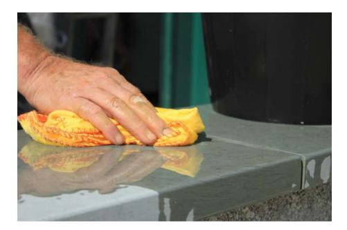
Using the techniques as described above, continue to lay all the coping stones until complete. Be sure to continually check the levels with a spirit level. Mortar spills can be a common occurrence during coping stone installation. Have a bucket of clean water and sponge close to hand and clean up any mortar spills immediately as they happen.
