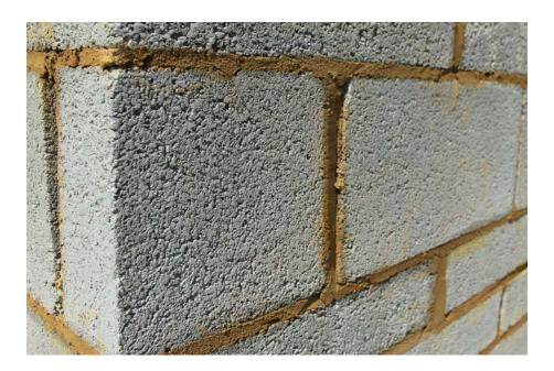
Good preparation is key to the success of any coping stone installation. Walls should be constructed using concrete blocks and built on top of strong concrete foundations. Walls should also be flat and free of any protruding mortar. If possible try and design the walls to dimensions that minimise the number of cuts to be made to the coping stones. Any cavities should be filled with concrete or compacted DPt (MOT) Type 1.
