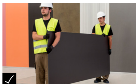
✓ When the ceramic slab is in a vertical position lift it, keeping it always upright.
