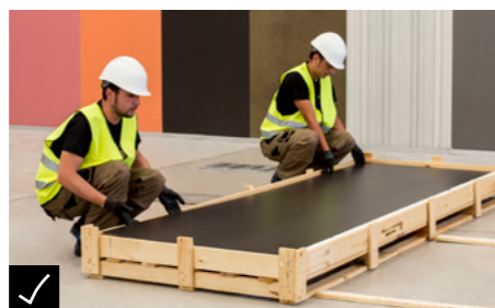
✓ The 1500x1000mm DesignClad slabs must be removed from their box by two people situated in parallel.
