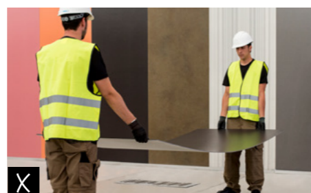
✗ Do not hold or transport the ceramic slab in a horizontal position.
