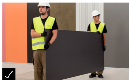
✓ When the ceramic slab is in a vertical position lift it, keeping it always upright.
