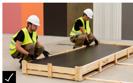
✓ The 1500x1000mm DesignClad slabs must be removed from their box by two people situated in parallel.
