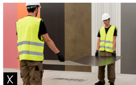
✗ Do not hold or transport the ceramic slab in a horizontal position.
