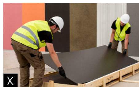
✗ Do not remove the ceramic slab holding it by the corners.
